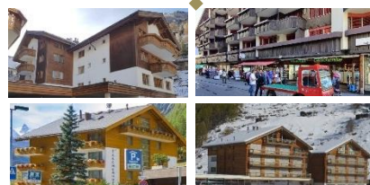
Commercial and residential properties in Zermatt/Täsch
